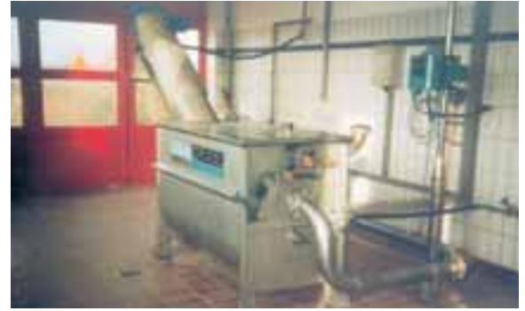
Indoor installation of a ROTAMAT® Sludge Acceptance Plant
