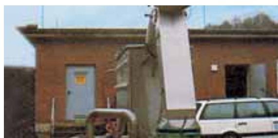
Bagging unit for the screenings
